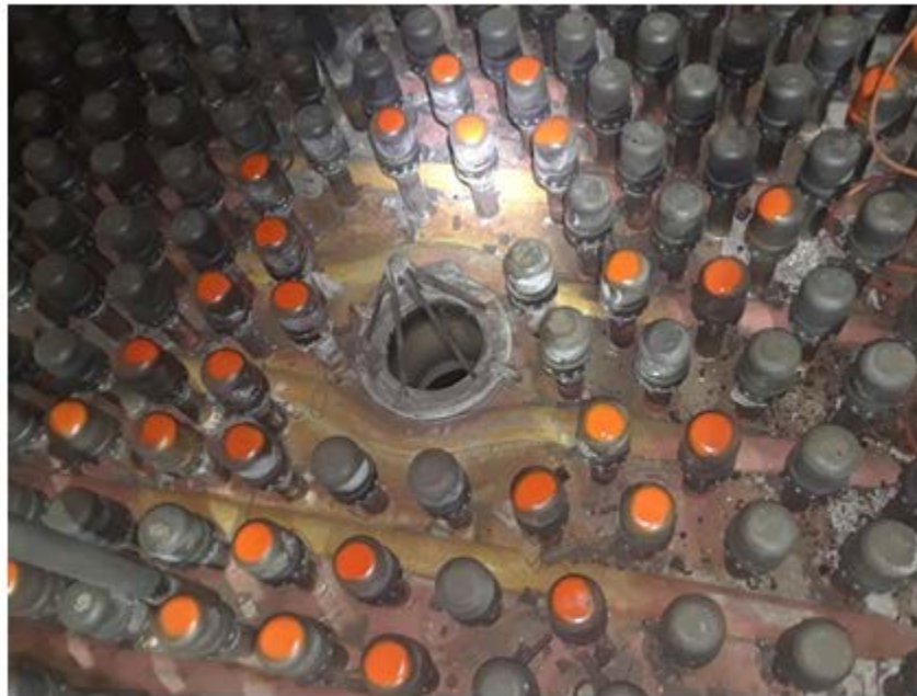
Pic 1: Furnace Bottom with rows of air nozzles surrounding one of the four bottom ash outlets that has been fitted with a simple "Witches Hat Strainer". For reference, the outlet pipe is 12" in diameter. The "Witches Hat Strainers" are five \frac{3}{4} " thick, 16" long stainless bars welded together to form a teepee.
