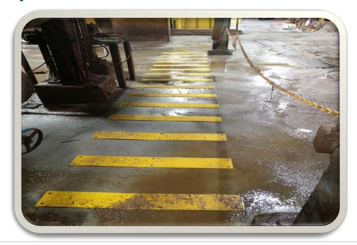
Removed vertical ladders and added stairs to the pulper area as well as throughout the mill.
