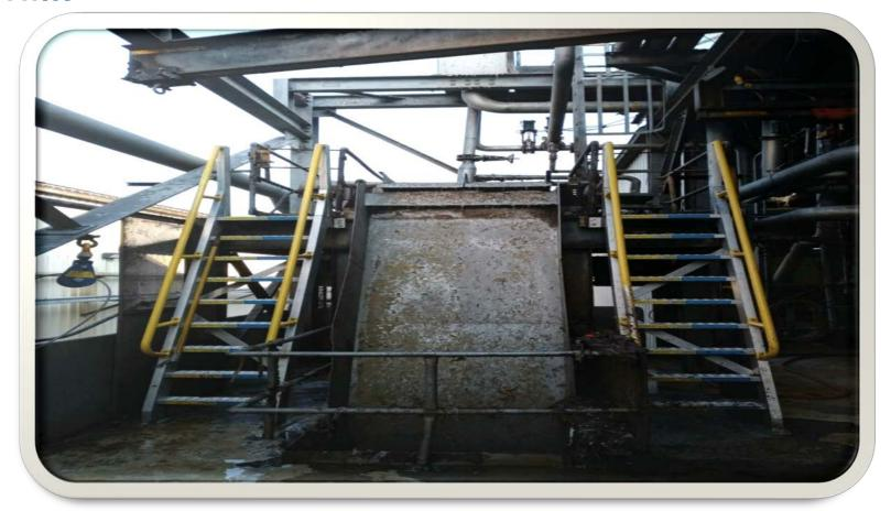
Added cable system to help with the ragger tails on top ply; now operator is out of the line of fire, reduced LCE possibility.
