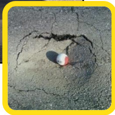
Asphalt Sinking
