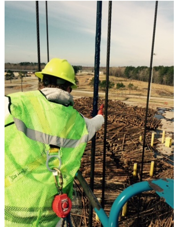
Grease applied by hand
