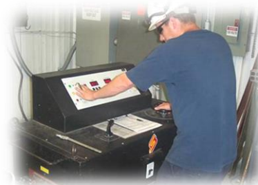
Primary Injection Testing
