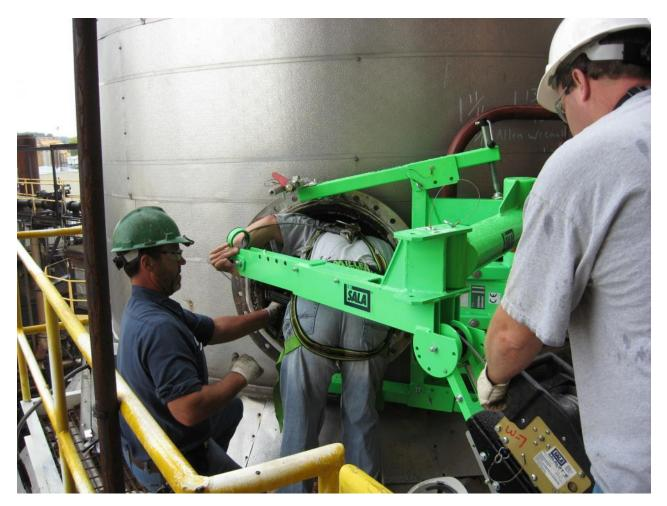
Employee in space, standing on scaffold plank attached to retrieval device which is also an SRL
