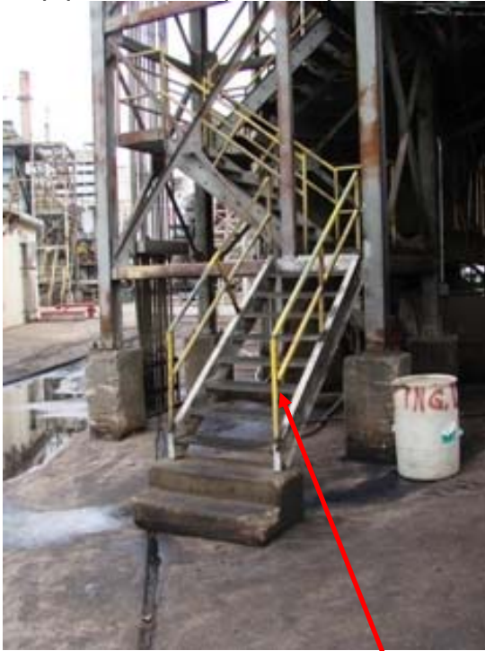
Location of incident. Note handrails stop. Handrails extended. Still will repair/paint concrete.
