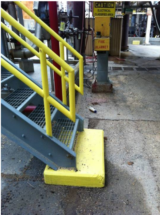
Single-Step Concrete pads will be painted yellow with non-slip surface.
