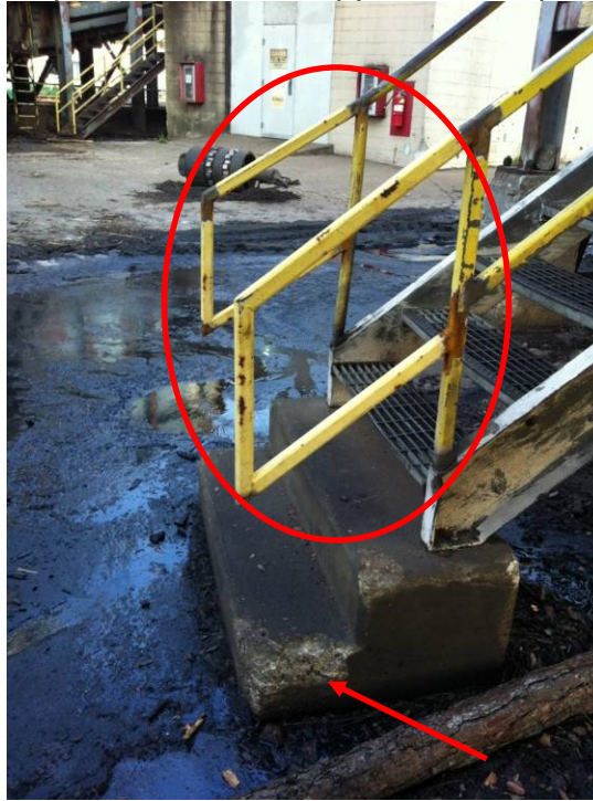
Location of incident. Note handrails stop. Handrails extended. Still will repair/paint concrete.
