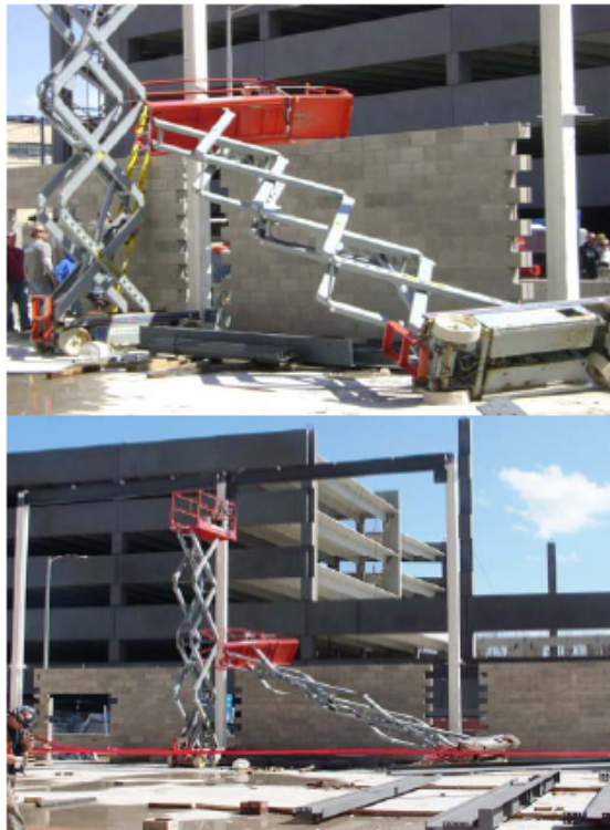
Picture of the complete work area with lift blown over.
