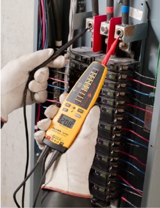
Figure 2. For your second test, pick a digital, not solenoid, electrical tester.
